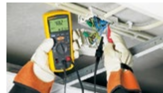
Wiring test in a small distribution box – all in one spot
