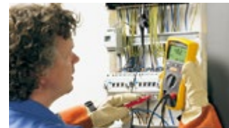
Insulation test at a distribution panel
